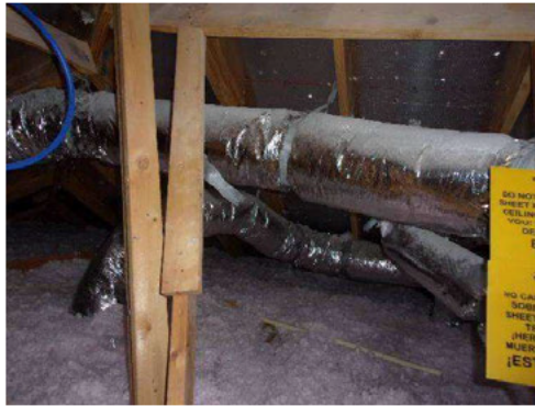
Attic (w/radiant barrier)
